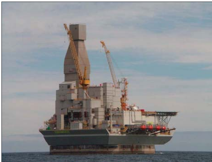
The Orlan platform, operated by Parker Drilling crews, was used to drill extended-reach targets off the coast of Sakhalin Island for the Sakhalin-1 Consortium. (Fig. 1; photo courtesy of Exxon Neftegas Ltd.)
